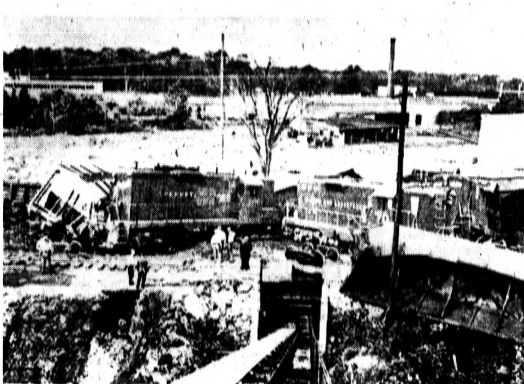
FREIGHT TRAIN COLLISION — When two freight trains collided on Kalamazoo's south side this morning, 10 empty cars were derailed, and three heavy diesel engines were heavily damaged. Five trainmen escaped in-
