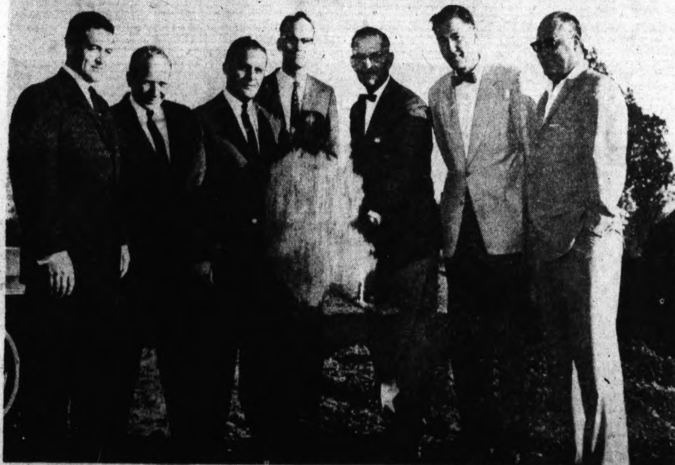
HEAVE HO—Mayor Robert Landry heaves the first shovel of dirt at the official ground breaking yesterday for Pontiac's new water plant. Participating in the ceremony are (from left) Commissioners William H. Taylor Jr., Loy L. Ledford, Winford
