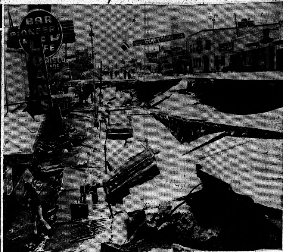
Once level, this three-tier Anchorage street typifies the damage caused throughout Alaska by the continent's greatest earthquake. Fishing fleets, industry, rails and thousands of private homes—60 per cent of the state's developed worth—were left in wreckage. Toll was 130. Tremors rocked West coast cities southward as far as northern California and huge 'quake spawned tidal waves pounded across the Pacific to damage Hawaii.
