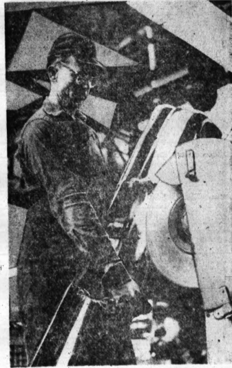
BUFFER — This Pontiac rear bumper is light enough so that Eugene Lamberson, 575 Second St., can hand buff it on a power wheel. Lamberson works in the chrome plating plant.
