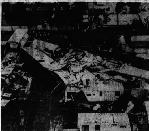
TWISTER TOPPLES TRAILERS — A tornado hit a trailer park near Fort Lauderdale, Fla., yesterday, damaging and overturning the wheeled homes and injuring at least six persons. The twister was one of six that hit south Florida. Damage to communities was estimated at $500,000.
