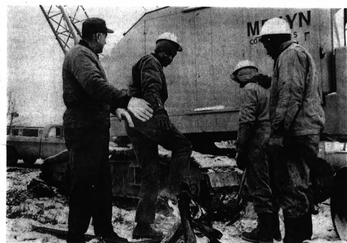
HOTFOOT — Construction workers at M59 and Elizabeth Lake Road in Waterford Township wasted no time this morning in lighting a fire to keep warm. When they arrived on the job, the temperature was at a low of seven degrees.
