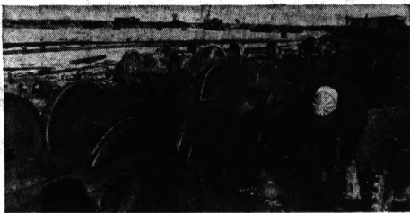
A torchman works on a wheel assembly, breaking it down to movable size.
