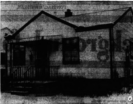
SMALL HOUSE — This is the Derrell Kelley home at 235 West Fairmont street about three weeks ago. Attractive and well kept, it was bit small for a family of five. More bedrooms
