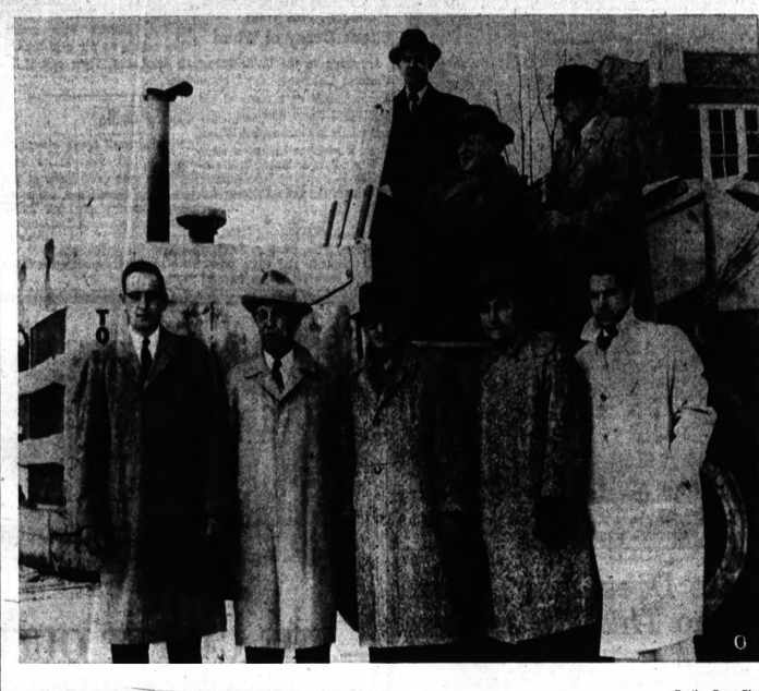
AT GROUND-BREAKING CEREMONY —Officials of neighboring communities were on hand yesterday for the ground-breaking ceremony for a new $93,500 Michigan Bell Telephone Co. branch office in Waterford Township. Along a huge tractor are State Rep. Lloyd L. Anderson (R-Waterford Township); State Sen. L. Harvey Lloyd (R-Oakland County); and Raymond H. Storm, district manager for Michigan Bell. Standing in front of the tractor are (from left) William B. Taylor, Sylvan Lake mayor; John C. Rehard, West Bloomfield Township supervisor; Edward Douglas, Orchard Lake Village commissioner; Elmer Johnson, Waterford Township supervisor; and Vern Taylor, Keok Harbor road supervisor. The surrounding communities represented will also benefit from the new branch to be built at Cass-Elizabeth Lake and Hogarth roads.
