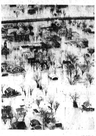
ISOLATED TOWN — Shepherdsburg, Ky., stands partially under flood waters of the Ohio River and its tributaries yesterday. In the downtown district, water averaged seven feet deep. The town was isolated, and other nearby communities were evacuated.
