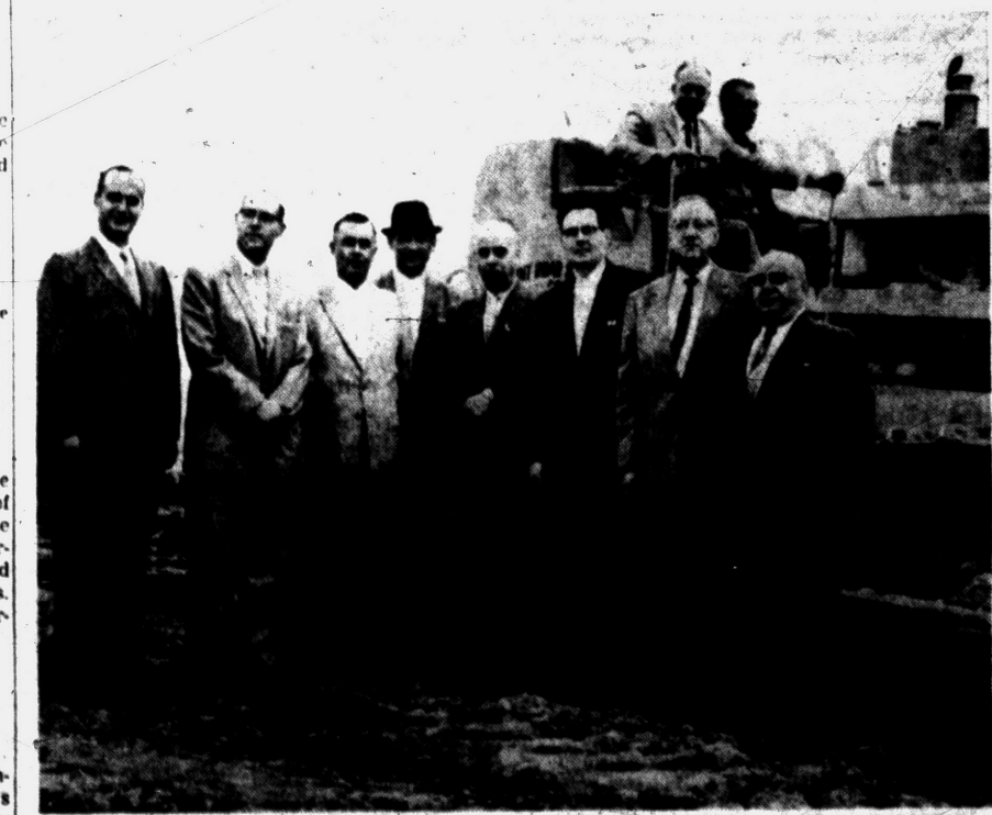
AT DRIVE-IN GROUND BREAKING — A large group gathered as bulldozers began leveling ground for the new Miracle Mile Drive-In. With a construction man in the cab of the bulldozer is Eldon Samuels, owner of the new theater. Others at the ceremony are (from left): Grant Silverfarb, Louis Silverfarb, Karl Rhodes, Bernard Edelman, Arno Hulel, Leg Sadowski, Clarence Williamson and Benjamin Lefkowitz.
