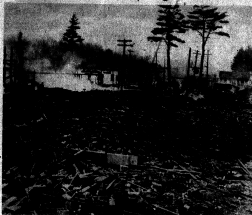
FIREWORKS PLANT DESTROYED — This is a general view of the ruins of the main building of the Rockland Fireworks Co., of Randolph, Mass., which was destroyed by explosions yesterday. In the background are other buildings of the firm, which were damaged.
