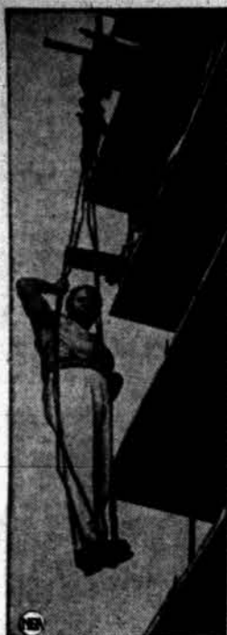
GOING UP — Col. Terrell J. Murrell rides hoist to inspect his apartment building.
