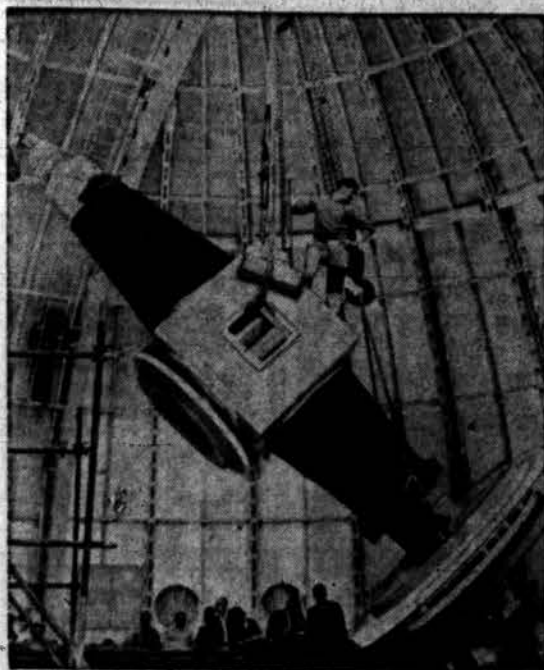
THE BIG EYE —The giant axle of the world's second largest telescope is ridden into position by a construction worker high above the floor of the observatory at St. Michel de Provence, France. The 1½-ton mirror for the telescope is being completed in Paris. When finished the big eye will be second only to the telescope at Mount Palomar, Calif.
