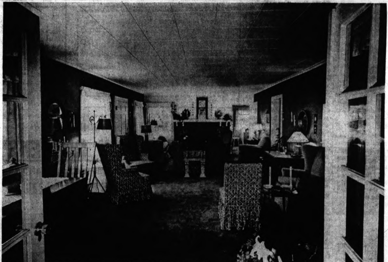
Double Doors Lead From The Porch Into The Formal Living-Dining Area
