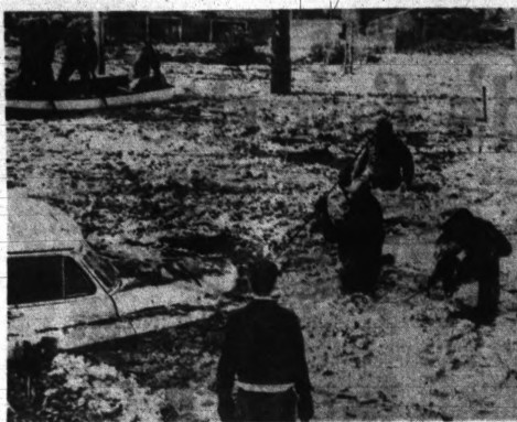
WATER, WATER EVERYWHERE — St. Louis suffered from too much water Wednesday when a huge water main broke in a northern section of the city. In picture on the left, city employees are up to their waists in cold water trying to break the ice from frozen manholes in an effort to let the water drain out. The
