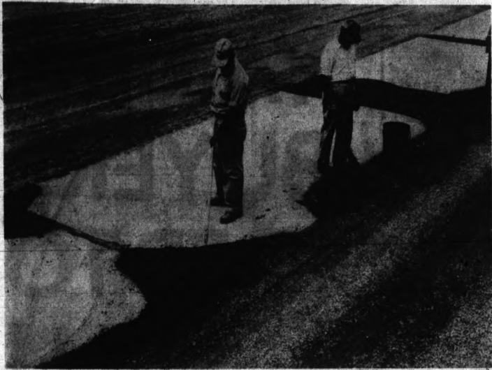
BUILT-IN BUMPS — Here General Motors Corp. construction workers go to work on a new road at the GM Proving Grounds near Milford — mauling it up. The men built in every type of
