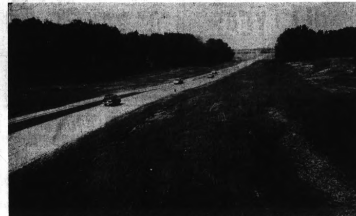
A SAFER HIGHWAY — Tomorrow's highways may look like this, where every roadside hazard has been eliminated for a distance of 100 feet on either side. The improved road has been built
