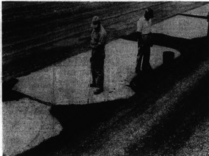
BUILT-IN BUMPS — Here General Motors Corp. construction workers go to work on a new road at the GM Proving Grounds near Milford — messing it up. The men built in every type of
