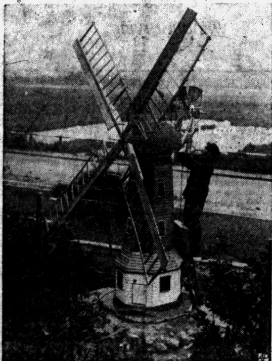
ALL FOR LIGHT —Richard Brauer evidently believes in harnessing the elements for his lighting source at Hamburg, Germany. He built this windmill to drive a generator which will make electricity to light his garden.
