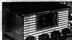
A ROOM ADDITION
