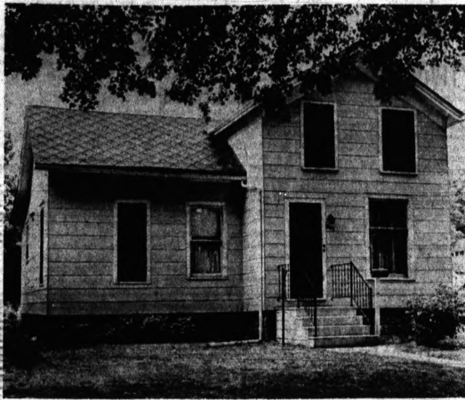
NEW EXTERIOR — Mrs. Gloria Lagasey, 154 Judson, has about completed improving the exterior of the 4-family house she owns. Aluminum siding updated its appearance. The old porch was torn off and a new one built. Inside there is a new furnace and the plumbing is scheduled for over-hauling. Both owner and Urban Renewal authorities are proud of the job.
