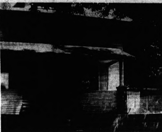
OUT-OF-TOWN OWNER — Oliver Lawson of Temperance, Michigan is the owner of this 2-family house. He was discouraged by poor tenants in the past and the deteriorating condition of the neighborhood. But he went along
