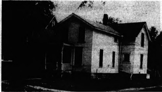
MULTIPLE-FAMILY —This rambling house at 154 Judson is owned by Mrs. Gloria Lagasey. It houses 4 families. When inspected by Urban Renewal authorities, they found it in good shape. But the owner wanted to make some improvement. See the house as it appears today
