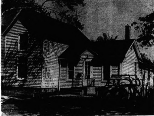
191 CHANDLER — This house owned by the Leon Putmans, was originally slated for acquisition in urban renewal, but plans were changed. After removing 3 huge trees that shaded the house too much, the Putmans repainted and started interior improvements. Putnam, partially disabled by a stroke 4 years ago, is doing all the remodeling himself. Already there is a new gas furnace, a completely new tiled bathroom and new paneling in the den. Kitchen remodeling comes next. When the Putmans bought this house 25 years ago, it was already old. They remodeled it then.
