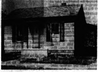
MUST BE SEEN —If you compare this picture with the "Before" shot above you'll find it hard to believe both are the same house. The John R. Lumber Company of Madison Heights completely rebuilt the interior of this 3-room home. Inside it is clean and shining and safe. Outside, it is a credit to the neighborhood. About the only things left are the sturdy basement and the little side porch (even that was jacked up). The house is at 60 Parkhurst and is for sale.
