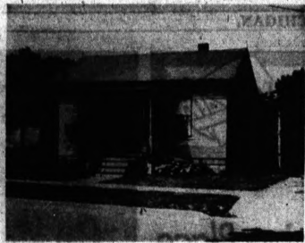
AN EYESORE —The neighbors were unhappy with this little old house on Parkhurst. It was shabby and run-down. Urban Renewal authorities acquired it. Then the John R. Lumber Company of Madison Heights stepped in and spent over $5000 on the house. See the "After" picture below.
