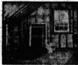
BEFORE —Shows just before remodeling started, old attic was useless. Now double-hung windows of ponderous pine replaced single sash for more natural light and good looks.
