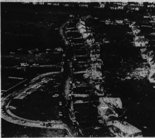
TWISTED NEIGHBORHOOD — This aerial view shows the Overland Park, Kan., neighborhood which was struck by a tornado yesterday. The funnel skipped by the elementary school at left and hit the homes across the street. An estimated two dozen homes were destroyed or damaged.
