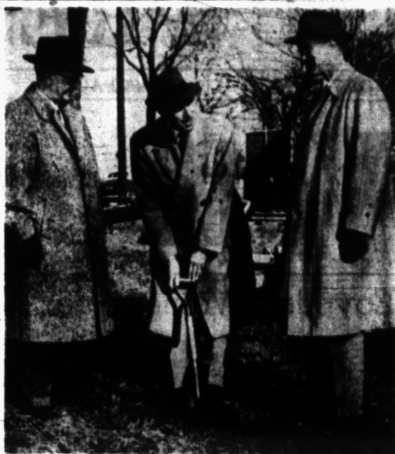
FIRST SPADEFUL —Land was broken for the new $100,000 Automobile Club of Michigan office at 250 S. Hunter Blvd. yesterday by club President Clarence Otter, center, of Bloomfield Hills. Douglas Brown, right, manager of the Pontiac AAA office since 1946, will direct the new office, which will serve the 7,000 club members in the Birmingham area when completed July 1. Assisting is club General Manager E. S. Matheson, left. Also present were club directors John A. Brown and Roy M. Hood of Birmingham and James M. Verner of Bloomfield Hills.
