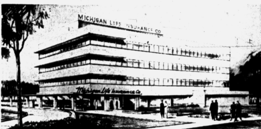
GROUND BROKEN — Work has begun on the new four-story $1,100,000 office building of the Michigan Life Insurance Co., to be located on a three-acre site on the west side of Woodward avenue in Royal Oak, just south of Coolidge Road. Of modern design, the building will be completely air-conditioned, and faced with Indiana limestone. Facilities for a banking office of the Wayne Oakland Bank of Royal Oak will be provided on the first floor.
