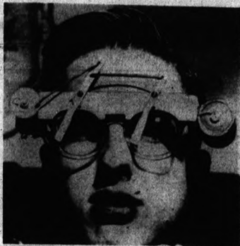
A MAN OF VISION — Donald Andrus, 17, devised this wiper assembly to keep his eye glasses cleared of snow and rain. A flashlight battery powers the device which is controlled by a lapel switch. Andrus tried it out in Wednesday's heavy snowfall in Rochester, N. Y., and he says it works fine.
