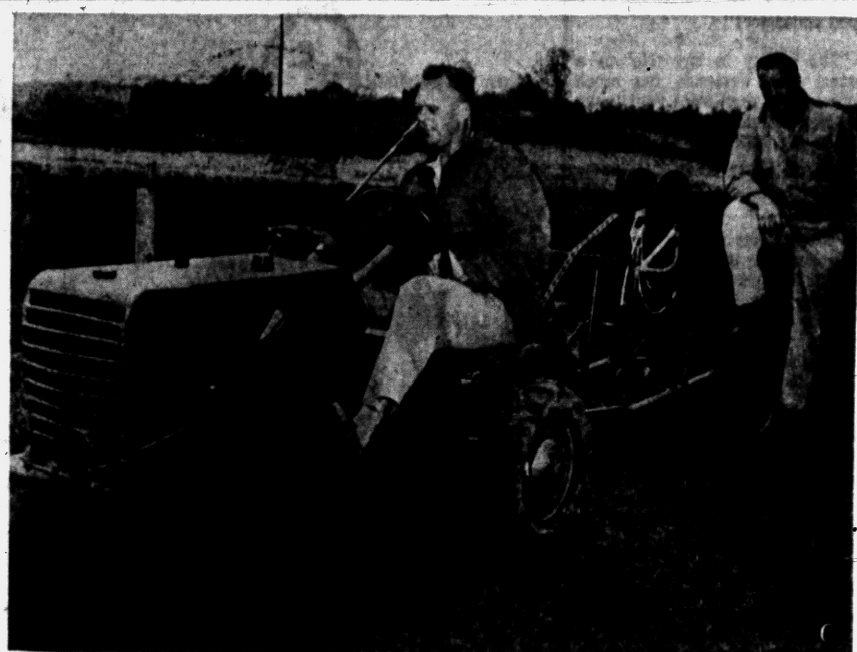
'LITTLE MONSTER' WIRE PLANTER — George Shoebridge lays electrical wire for the National Girl Scout Encampment at Haven Hill at the rate of one hundred feet in 90 seconds. He does it with a contraption of his own invention called a "wire planter." The planter is pulled by a specially-built tractor which he has dubbed "Little Monster."
