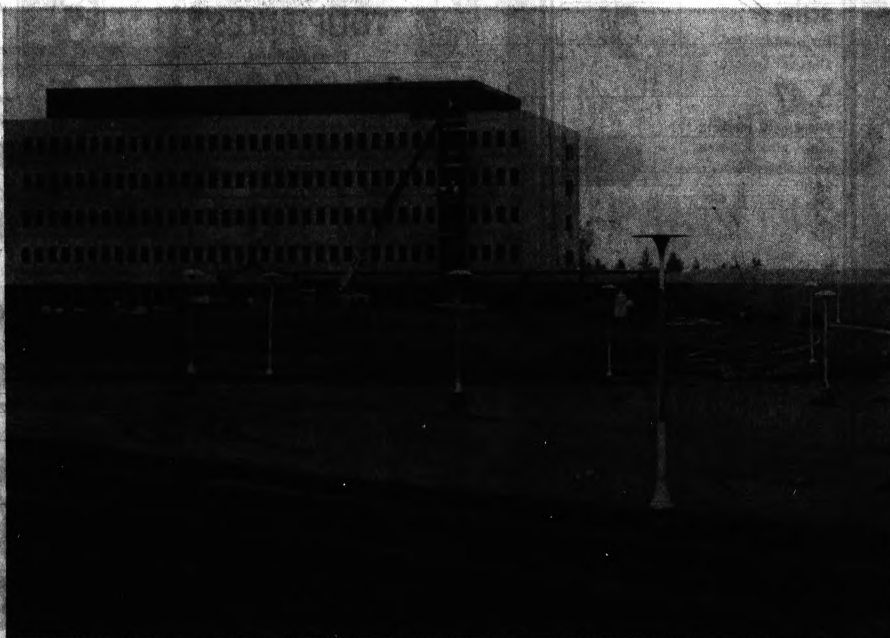
IMPRESSIVE STRUCTURE —The new Oakland Schools $3.3-million administration building is expected to be completed April 1. School officials
