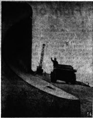
A WAVE CUTTER—Britain is remodeling the seawall at Dymchurch, Kent. Curved wall surface guides waves up and over to minimize pounding and undercutting.
