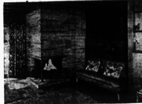
FIREPLACE FOR CORNER —Corner fireplace allows everyone in the room a good view of flames. This one is built around a double-walled metal form. Vents (visible above firebox) provide circulation of warm air.
