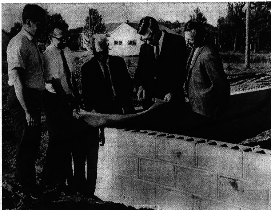
CHECK PLANS — Leaders of Good Shepherd Assembly of God go over building plans as they inspect the progress of the first unit of a new church under construction on Sashabaw, Independence Township. Shown (from left) are Arthur VanWagoner, 5200 E. Highland, Milford; Wes Wibley, 1600 Canton,
