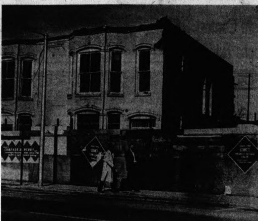
BEING TORN DOWN — Two substantial buildings, one wood and one brick on the east side of Rochester's Main Street, are being razed to make room for a used car lot. The demolition project by Kaverley Mercury Sales follows the village's example of tearing down old structures no longer fit for occupancy which included the old municipal building razed several weeks ago. The old Rochester hotel also has been condemned but its demolition has been delayed because of pending court action.
