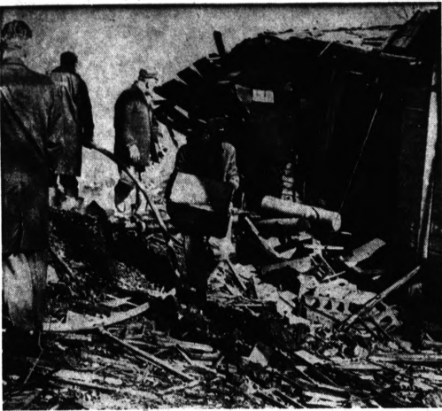
BLAST KILLS FIVE — Rescue workers probe the ruins of the Keystone Fireworks explosion killed five persons and injured Co. near Dunbar, Pa., yesterday after an several others.
