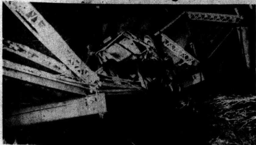
BRIDGE KNOCKED OUT —An automobile struck the west-central Wisconsin area. The car was wrapped around the steel girders of a bridge near Colfax, Wis., last night when a tornado was bent double.
