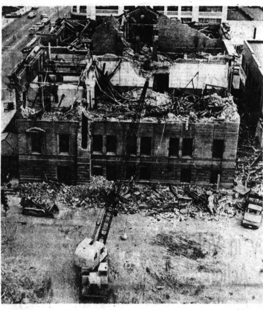
CRUMBLING COURTHOUSE — From top of the Riber Building, corner Wayne and Huron streets, the camera looks into the vanishing Old Courthouse. The large room laid open in front was a courtroom, with a judge's chambers at left. Chambers and court are separated by a wall and white-columned portico still standing where once the judge's bench was.
