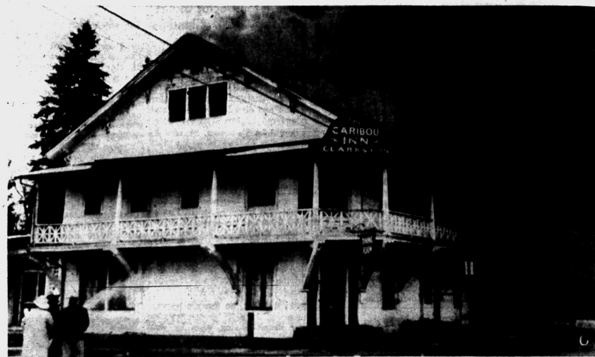
CARIBOU INN BURNS — Smoke pours from the top floor and through the roof of the Caribou Inn at Clarkston early today as firemen battle a blaze which gutted a part of the old landmark
