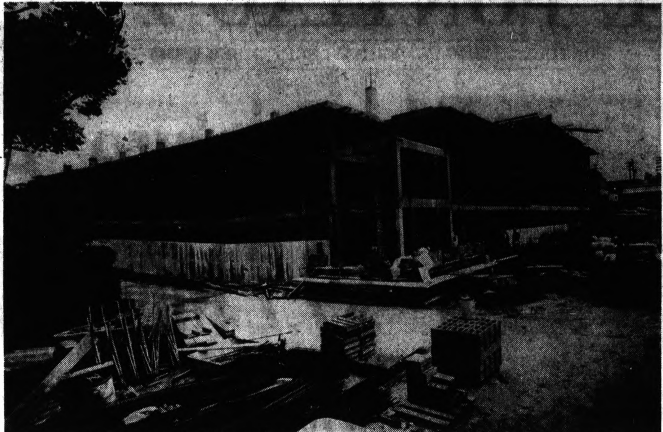
PARKING GARAGE—If work proceeds according to schedule, the City of Birmingham should have its first municipal parking garage completed by early next month. The facility, located on the corner of Woodward and Willis, will provide spaces for 566 cars on five parking levels. Construction work for the $1,016,000 structure has been under way since mid-February.
