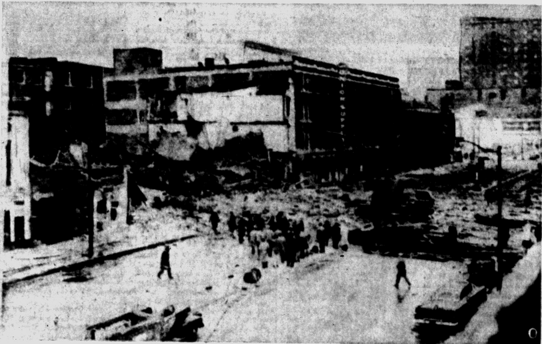
BUILDING DEMOLISHED —Completely demolished building above is where an explosion occurred today in Toledo's downtown business area. A wide area was rocked by the blast. One person is dead and a number still missing may have lost their lives.
