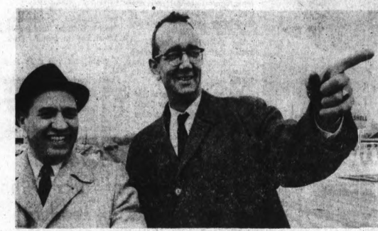
REVIEW ROAD PLANS — State Highway Commissioner John C. Mackie (right) and Waterford Township Clerk James E. Seeterlin discuss plans for the widening to five lanes of M59 from Elizabeth Lake Road to Airport Road as they view the highway near Elizabeth Lake Road. The project is scheduled for completion next year.
