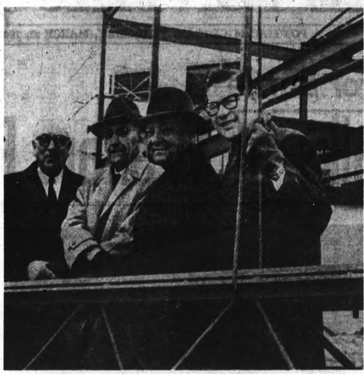
INSPECT BUILDING SITE — Civic and business leaders yesterday gathered at the Pontiac Mall to view the progress of a new two-story office and professional building being constructed. From left are A. C. Girard, president of the Community National Bank, which will have a branch in the building; Waterford Township Supervisor Elmer Jonhon; developer William Gersabson; and architect Arnold Agre.
