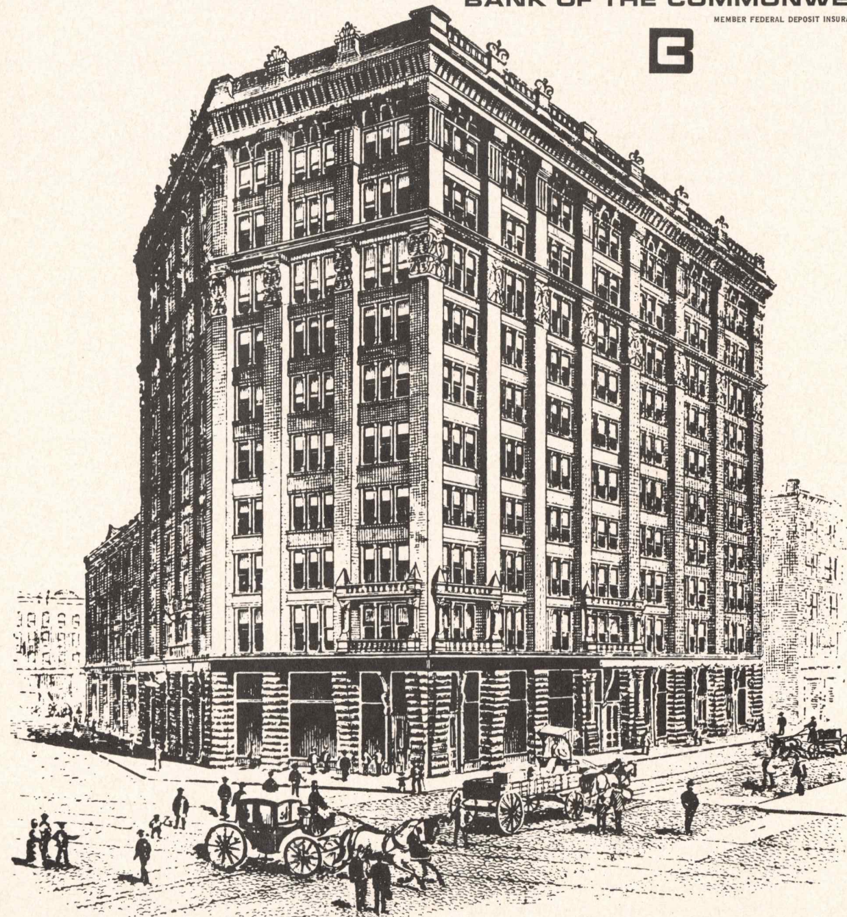
OUR FIRST HOME Original Bank of the Commonwealth, Hammond Building, Corner Fort and Griswold Streets. Courtesy Burton Collection, Detroit Public Library.
