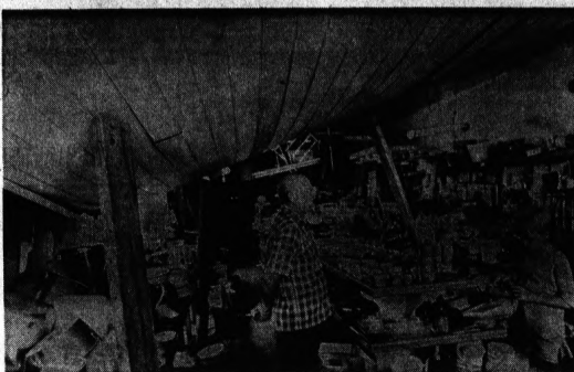
LOW OVERHEAD — Hardware dealer Alden L. Maufray (center) conducts business as usual despite a sagging ceiling that was propped up after a visit by Hurricane
