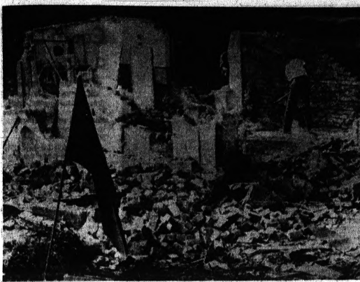
WRECK BORDER BUILDINGS — East Berlin homes near the border of West Berlin are demolished following the forcible evacuation of the residents by Communist East German police.
