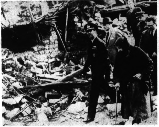
KING SURVEYS QUAKE DAMAGE —King Constantine of Greece walks through the rubble of a Megalopolis home destroyed by yesterday's earthquake, which left at least 17 dead, 200 injured and 30,000 homeless. A light tremor today caused fresh panic among the quake survivors. It brought down the ceiling and a wall of a church just before services were to be held for victims of the earlier quake.
