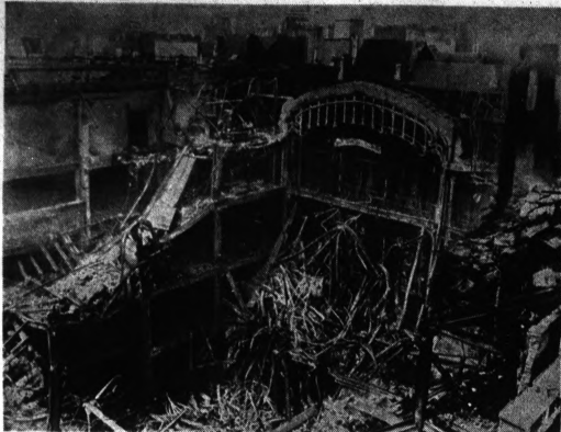
BRUSSELS STORE AFTER HOLOCAUST — This is a view today of the remains of the Brussels department store after fire broke out in the five story building Monday. Some 200 persons were reported missing and at least 13 persons were known dead.
