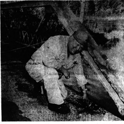
Public Works Supl. J. D. Caswell Examines Mont Eagle Bridge
