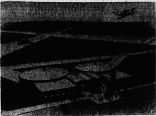
UNIQUE HANGARS — Two circular hangars, housing planes on a turntable, will be built at Lansing's Capital City Airport this spring. Gerald Francis, backer of the $400,000 project, said
