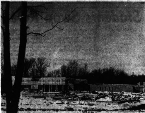
New Bloomfield Hills High School Under Construction
