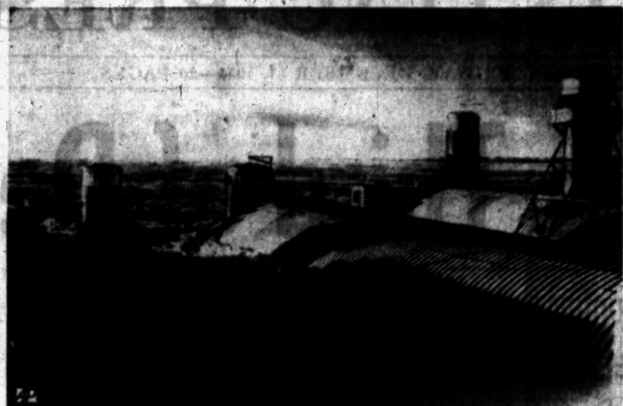
SINKING BASE BUILT IN GREENLAND —The Army released this photograph in Washington this week showing a new arctic military installation designed to sink slowly into the soft snow of the Greenland polar icecap. Buildings in foreground are steel tubes 18 feet in diameter. Vertical entrance towers are used. As the buildings sink, new sections are added to the towers to keep them above ice. Buildings are designed to sink several feet a year. Inside are quarters for several score Air Force men operating the weather observation station.
