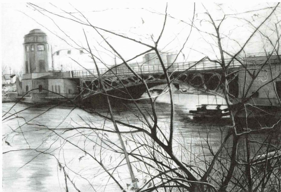
Fort Street Bridge, 2001 (reproduced in monochrome)
