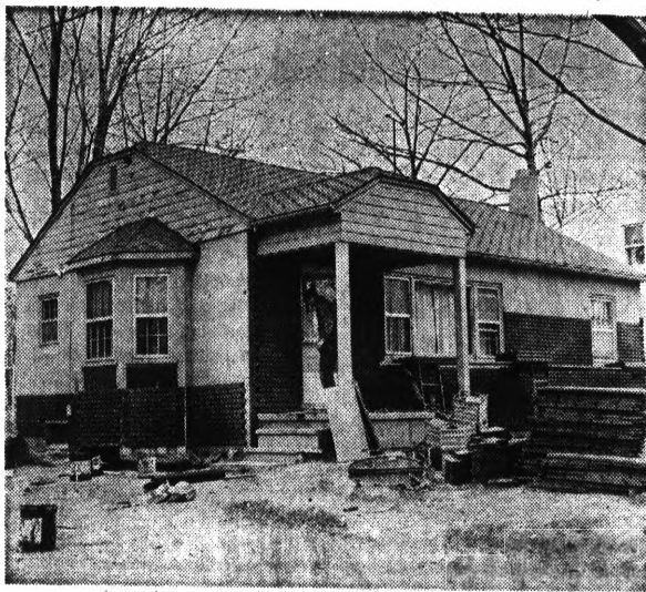
A face lifting that will be welcomed by you, your family, neighbors and the season. This job is being done by Klingelhut Brick Company.
