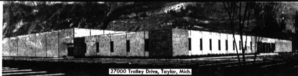
New home of RCA Distributing Corp. This gigantic distribution center is located near I-94 and Ecorse Road. The 64,000 square foot center contains display areas, offices, conference rooms and data processing facilities in addition to warehouse space.
