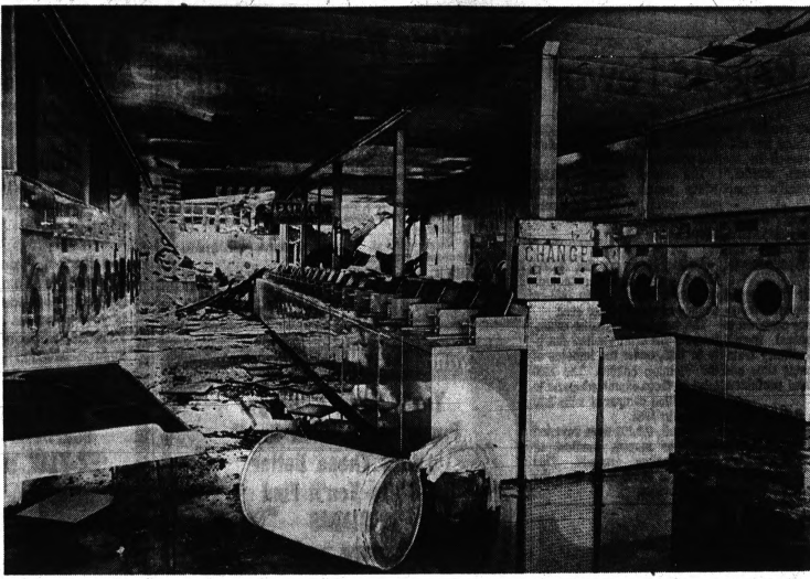
Debris Clutters The Romeo Coin Laundry Following Saturday's Fire
