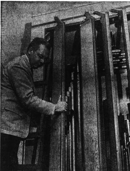
Continuous adjustment of the wooden louvers controls the expression of the pipes.
