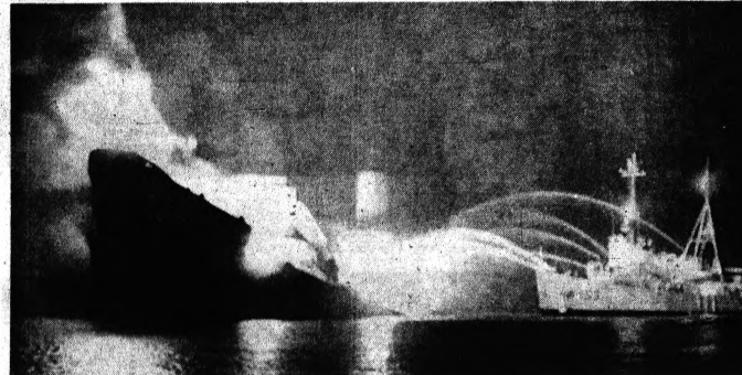
FIRE BOAT AT WORK —A naval fire boat plays streams of water on the burning naval tanker Potomac near the port terminal at Morehead City, N.C. The tanker, loaded with high octane gasoline and jet aviation fuel, burned through the night. At least one
