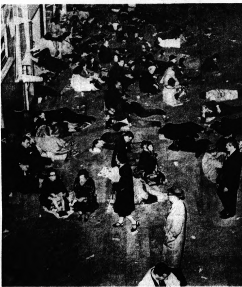
GRAND CENTRAL SCENE — This was the scene in New York City's Grand Central Terminal last night. Hundreds slept sitting up or lying down. This particular sector of the terminal was lit up with emergency lighting.
