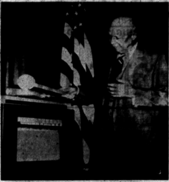
STARTS A-PLANT CONSTRUCTION—Waving a radioactive wand in a Denver television studio today, President Eisenhower started a shovel which broke ground at Shippington, Pa., for the nation's first atomic power plant for peaceful purposes. The President disclosed that the United States and some friendly countries are starting creation of an international atomic pool for peaceful use of atomic energy.
