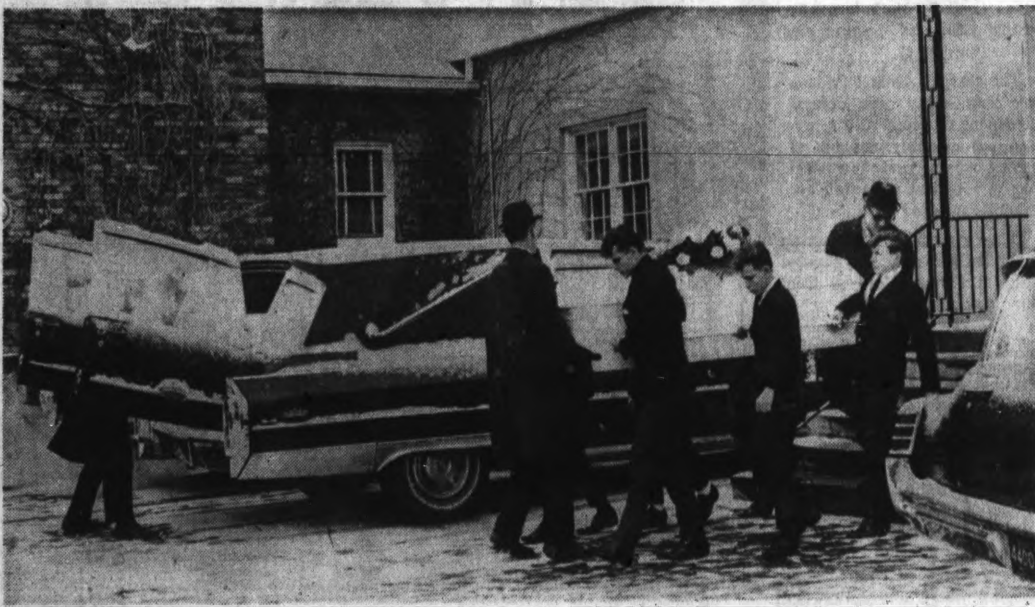
BROWN CHILDREN FUNERAL — Service for Mrs. Barbara Brown's four children, who perished in a house fire early Wednesday, was yesterday at the Sparks-Griffin Chapel. Killed in the blaze that raced through the frame house at 3980 Arcadia Park, Waterford Township, were Kathryn, 15; Nancy, 12; Donald, 9; and Julia, 7. The four children were buried at Waterford Center Cemetery after the 3:30 p.m. service.
